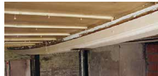
Apart from the improvement in airborne noise attenuation and fire protection, the Elascan TCC system also distinctly improves bending strength and vibration resistance.
